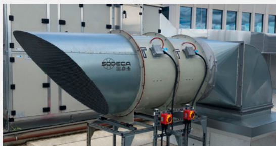
DEPRESSURISATION OF STAIRCASES Penrose Dock, Ireland
